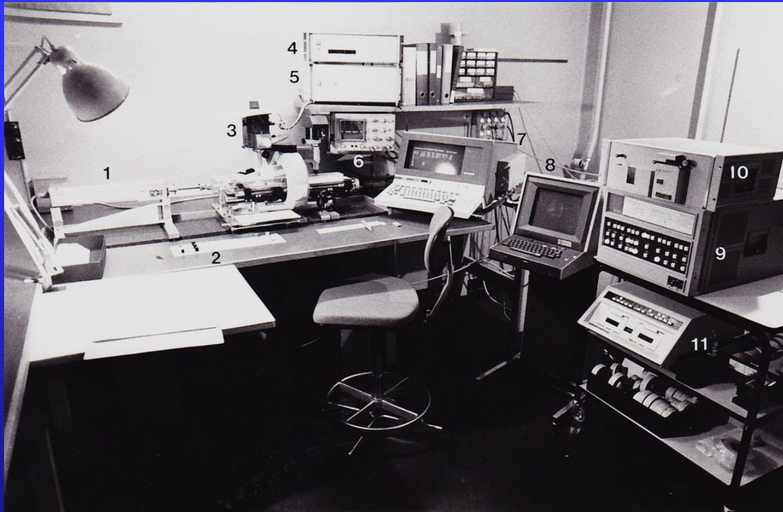
Modified Abbe comparator with line profile display & encoder
